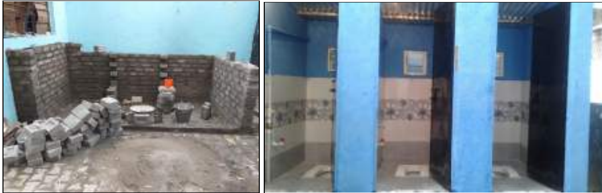
Toilet Construction completed at Synergy Pune Home
