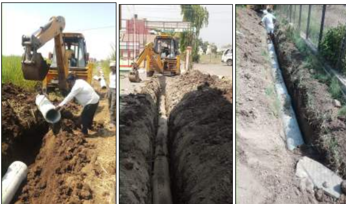
Excavation and laying of drainage pipeline: Vadhu Budruk Center
