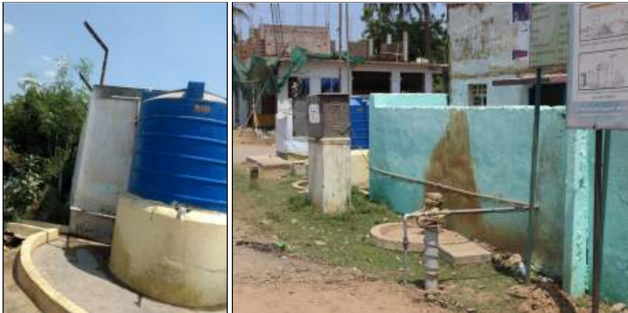
Water Supply Connections at Chithukadu Panchayat
